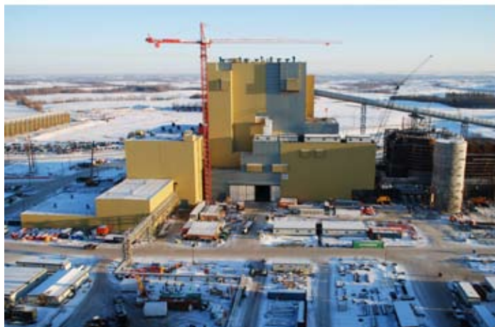
Construction of Keephills 3 (K3) – a 450 MW super-critical coal-fired plant
